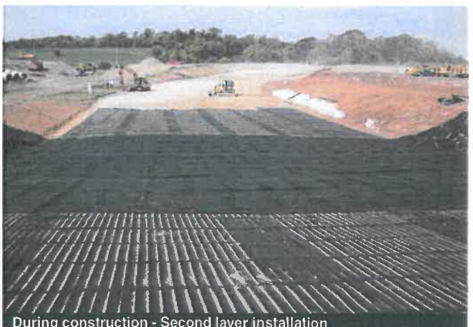
During construction - Second layer installation
