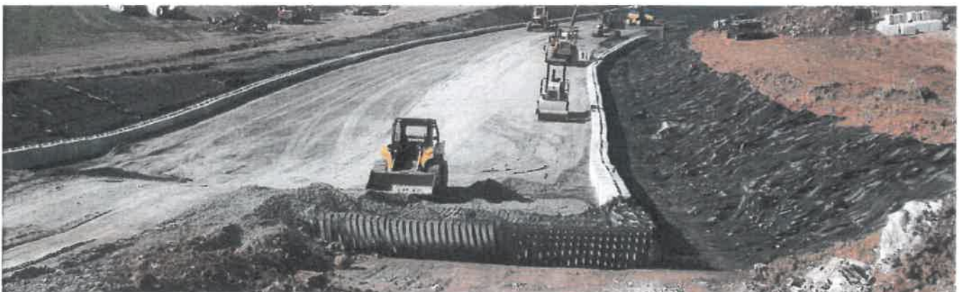
Basal Reinforcement Over Spanning Voids
