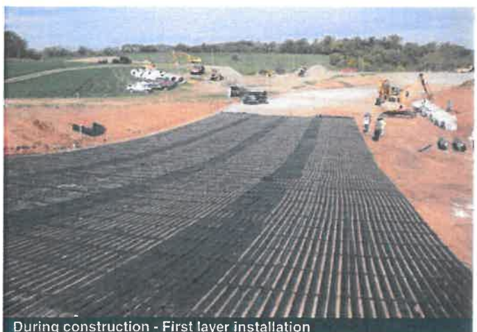
During construction - First layer installation
