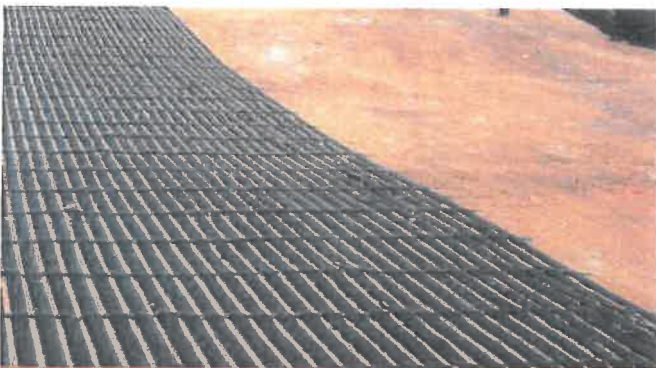
Close up a single direction installation of ParaLink®
